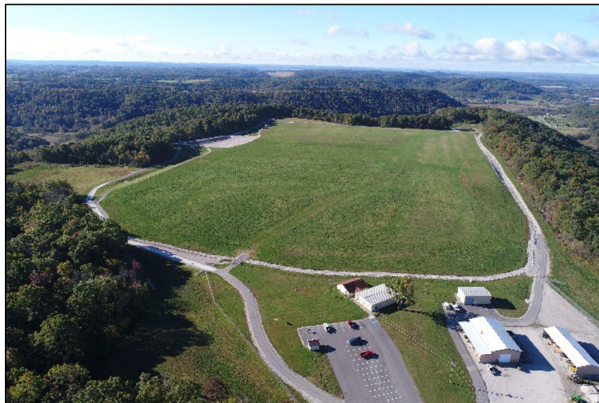
Photo 11: Maxey Flats, Post-Capping
