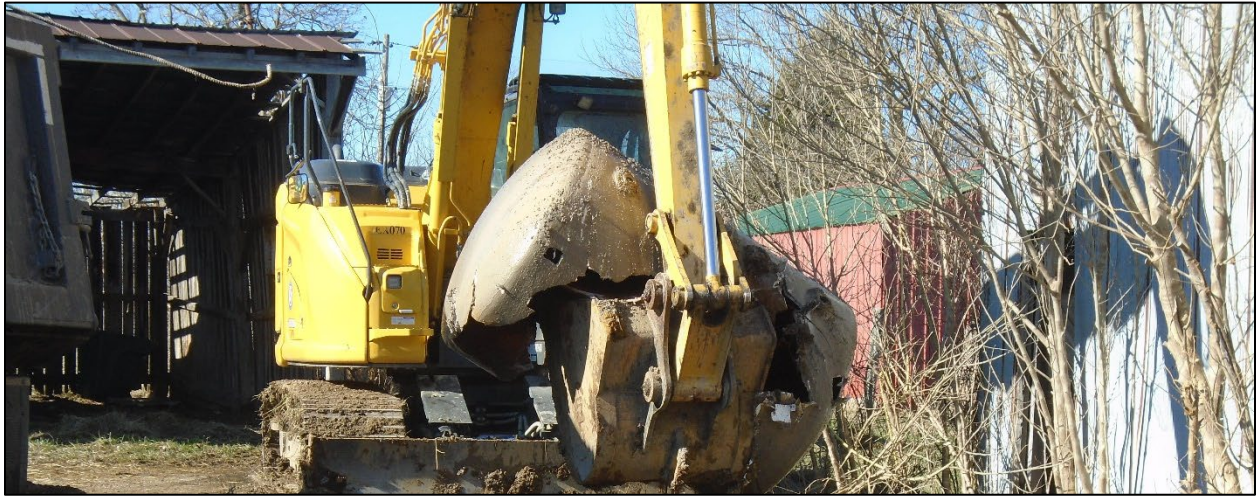
Photo 8: Removal of farm tanks at Rough River Youth Ranch
