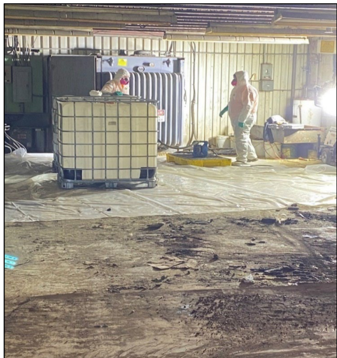
Photo 9: Kentucky Processing Prep Plant remediation
