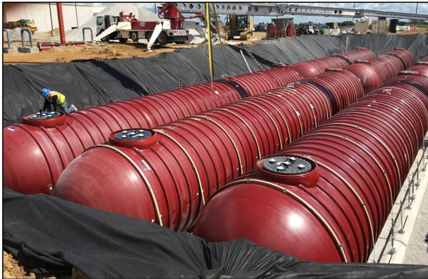
Photo 12: Underground Storage Tank Installation
