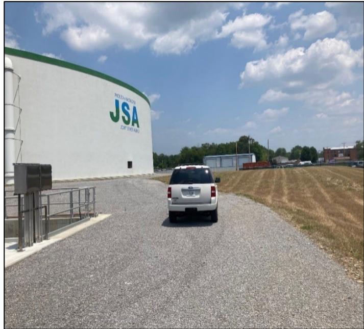
Photo 6: Paducah McCracken County, Joint Sewer Agency Tank
