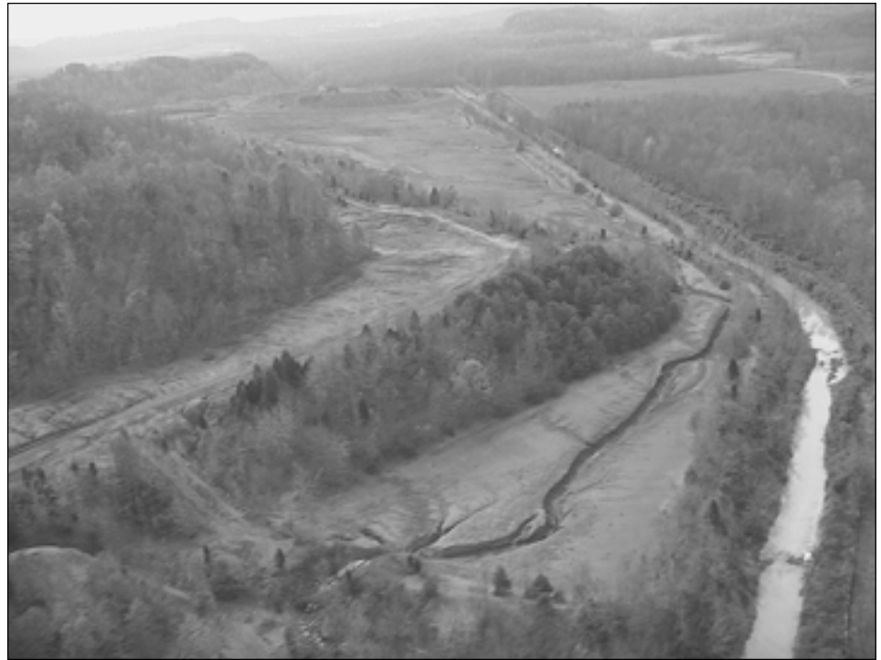
Looking upstream, barren acidic coal refuse and slurry along Pond Creek result in high metal and sediment loads. Nearly all of the material in the photo is proposed to be reclaimed as part of the Ebenezer project. Photo provided by the Division of Abandoned Mine Lands
