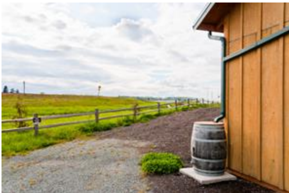
Above is a picture of a rain barrel collecting roof runoff
