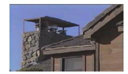
Chimney with Venting and Spark Arrestors - photo provided by www.firewise.org
