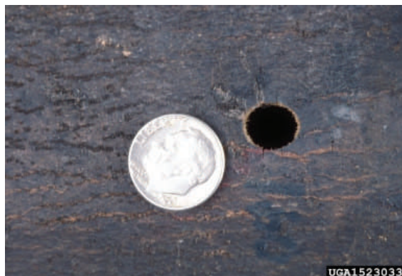
Figure 4. Redheaded ash borer exit hole
