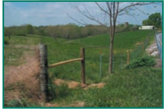
Figure 6. Cornerpost bracing on woven wire fence.
