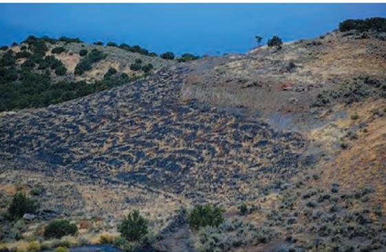
Construction at the fire occurred over an area of approximately 5 acres, and resulted in the excavation and quenching of approximately 168,000 cubic yards of material. The Skull Creek fire was completely excavated and cooled in approximately 7 months. Following replacement of the cooled material, the site was recontoured to natural slopes and revegetated.
