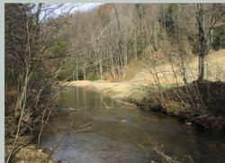
The Bear Hill Abandoned Mine Reclamation Project is located along the banks of the Casselman River in far Western Maryland. The project sealed two open mine entries, removed dangerous mining equipment and stabilized an eroding coal refuse pile. The coal refuse pile was being undercut by the river causing unstable stream banks and increased sedimentation. The photo shows the restored stream banks and newly graded site.
