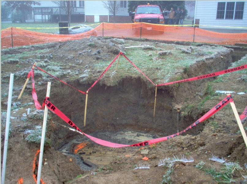
Subsidence, Midlothian, Virginia: Imagine waking up to see you backyard has subsided into a 1800s underground mine that you were never aware of. The Virginia Department of Mines, Minerals and Energy accomplished an emergency reclamation project to backfill the subsidence area, pour a reinforced concrete slab, topsoil and revegetate. (On the form)
