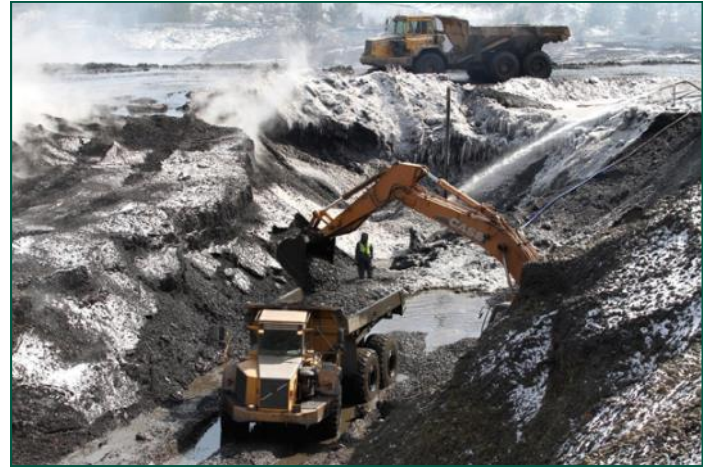
Temperatures fell into the single digits for almost a month while crews worked at Simpson Creek
