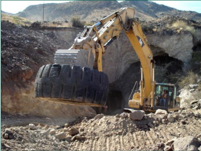
Crews placing used earth-moving equipment tires at Lake Valley.
