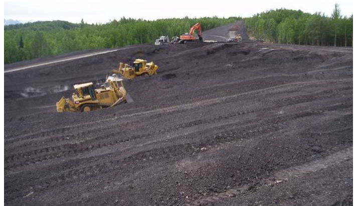
Figure 3 Mass production to prepare trenches for water flooding.
