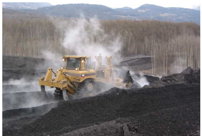
Figure 2 Jonesville Fire Phase II - Cat pushes trenches into hot refuse
