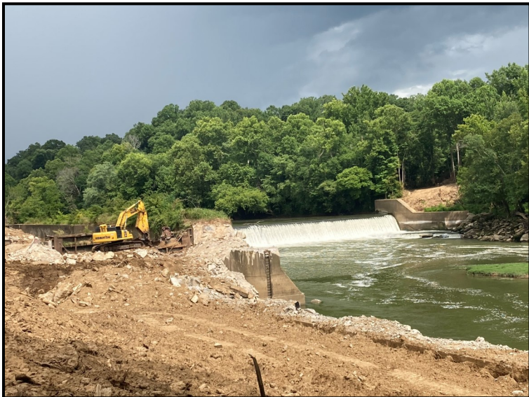
Demolition crews prepare the site for the removal of lock and dam #5.
