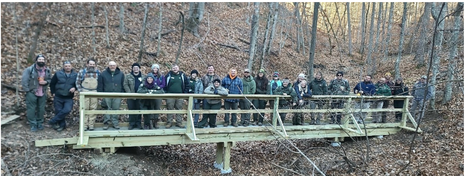
New 32 foot bridge built by participants of the OKNP Trail Workshop at Buckhorn Lake State Resort Park
