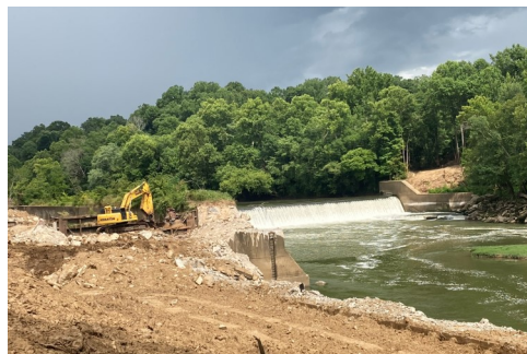
Green River, LD5 removal work
