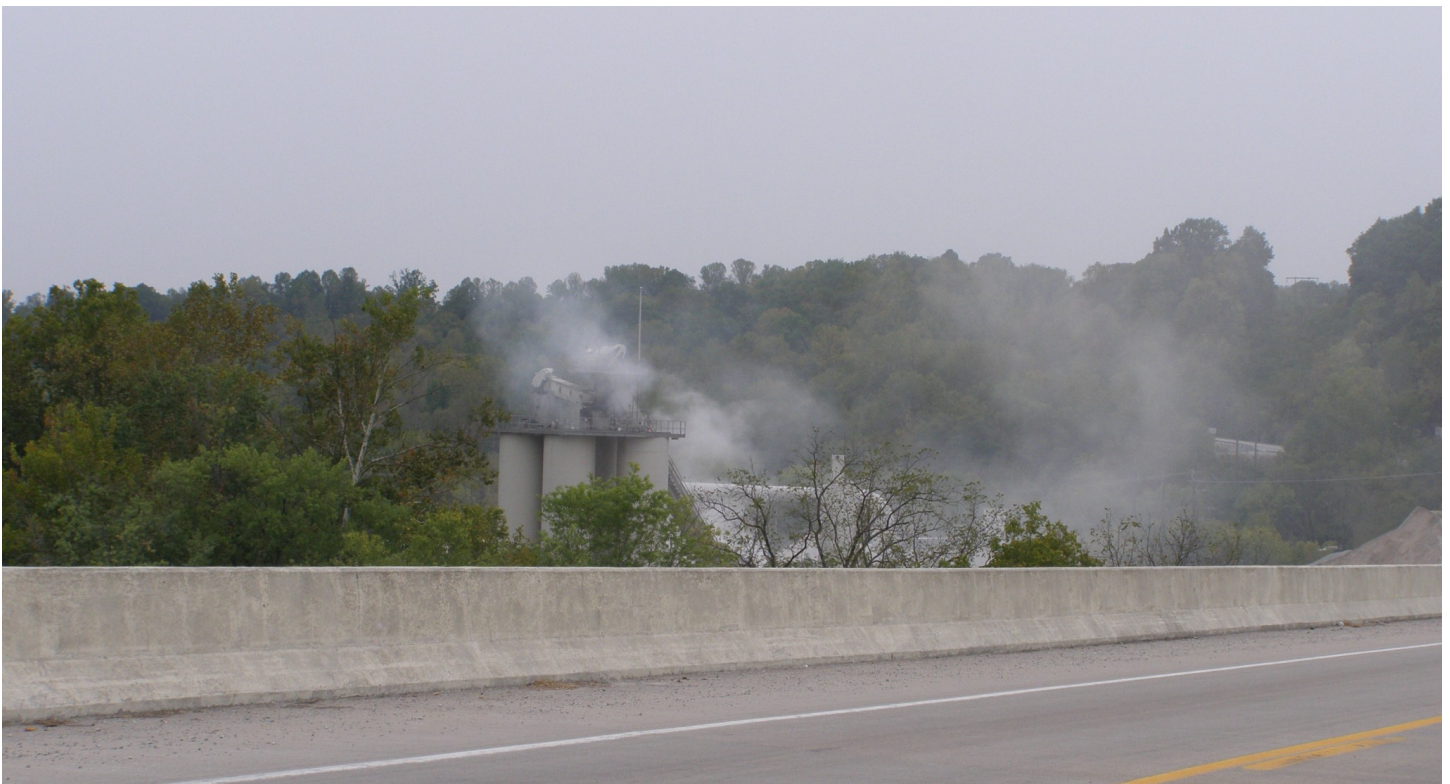
An example of fugitive emissions being released as dust from a cement facility. State regulation requires control measures such as spraying with water to reduce fugitive dust emissions and their impact on air quality. Photo: Division for Air Quality.
