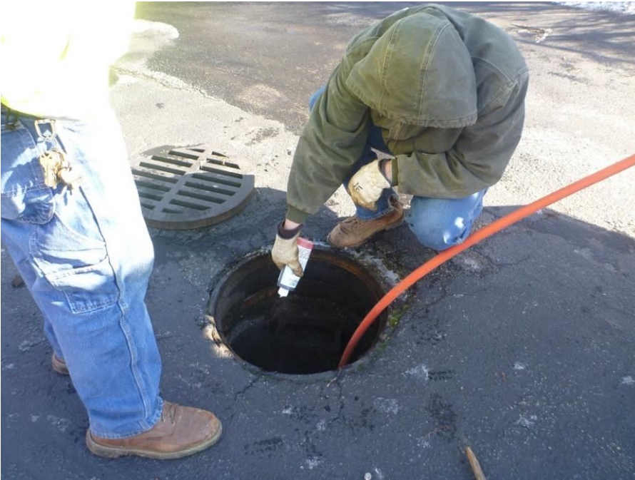
Figure 3: Dye Tracing City Sewers, Somerset KY
