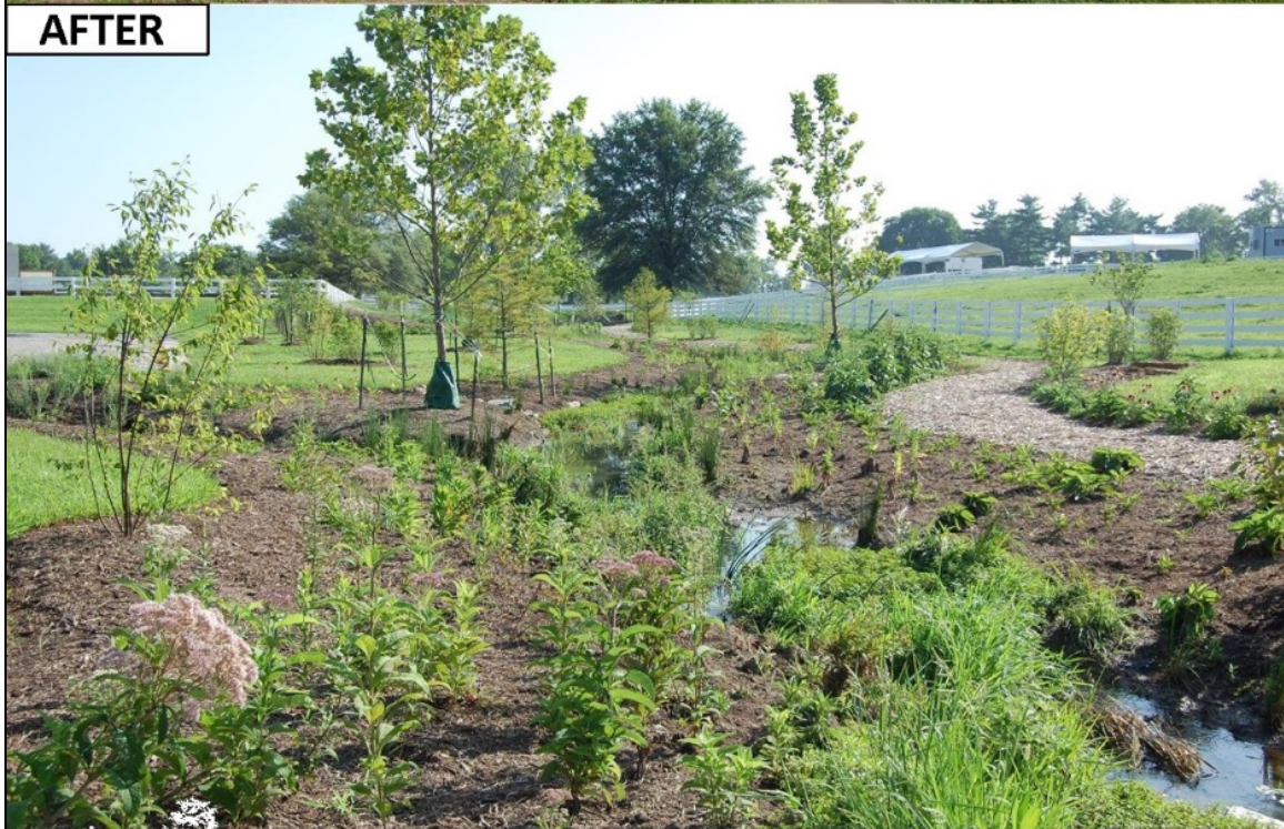
Riparian buffer at the Kentucky Horse Park, in Cane Run Watershed of the Kentucky River Basin, Fayette County, before and after implementation of best management practices outlined in the Cane Run Watershed Plan.
