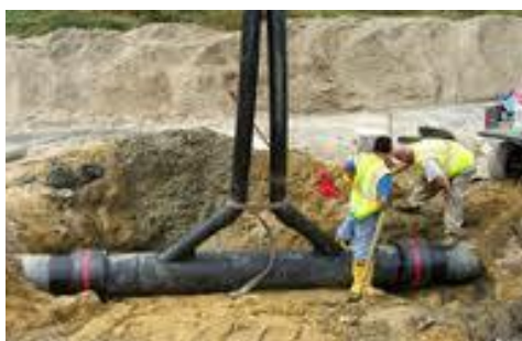
Picture 5-1 Pipe installation
