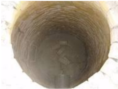
Picture 4-2 at left Brick manhole
