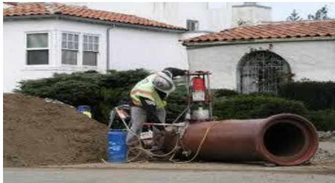
Picture 11-6 collection system rehab in progress
