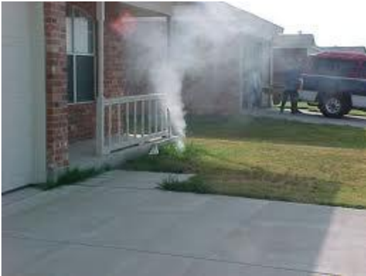
Picture 7-5 smoke testing
