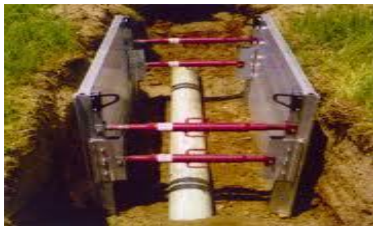
Picture 10-5 Properly constructed Trench box
