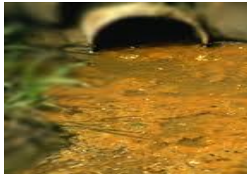
Picture 9-5 Sanitary Sewer Overflow from a grease trap
