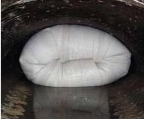
Picture 11-10 Cured in place pipe installation
