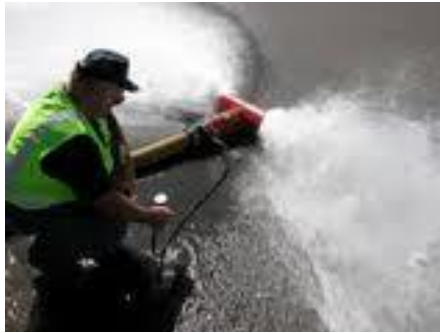
Picture 4-7 Line flushing
