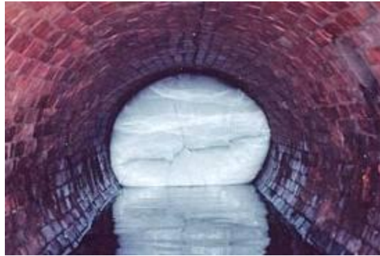
Picture 11- 12 fold and formed manhole rehabilitation
