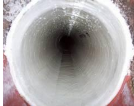
Picture 11-11 Cured in place pipe after installation
