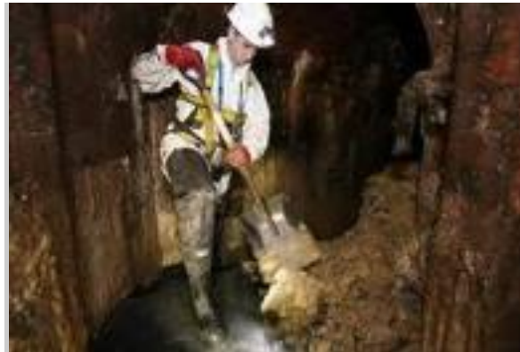
Picture 8-6 manual cleaning of a large sewer
