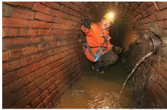
Picture 8-4 Operator inspecting a sewer.
