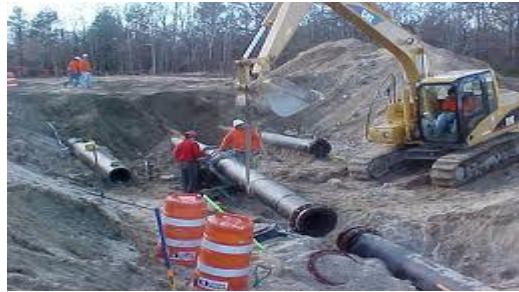
Picture 5-2 HDPE pipe installation
