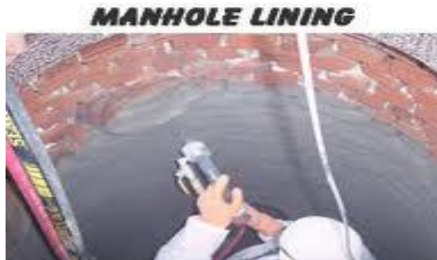
Picture 11-14 manhole being lined using spray trenchless technology
