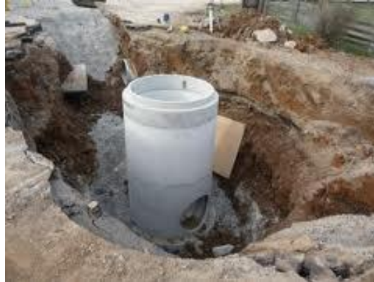
Picture 4-1 collection system installation
