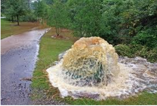
Picture 9-1 Combined sewer overflow
