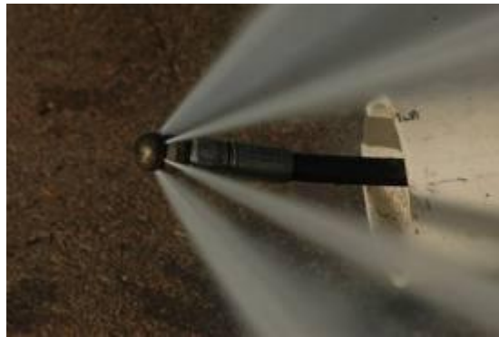
Picture 8-2 Jetting a pipe
