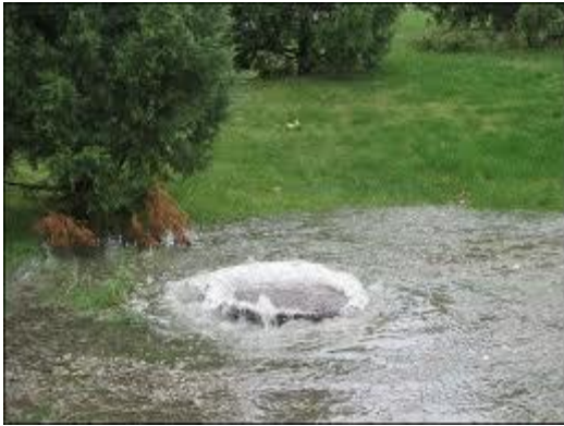
Picture 9-4 Sanitary Sewer Overflow from manhole
