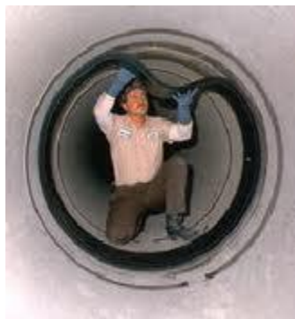
Picture 11-8 Internal pipe seal being constructed
