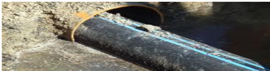
Picture 11-1 sliplining of a pipe
