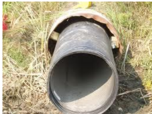
Picture 11-9 sliplining of a pipe
