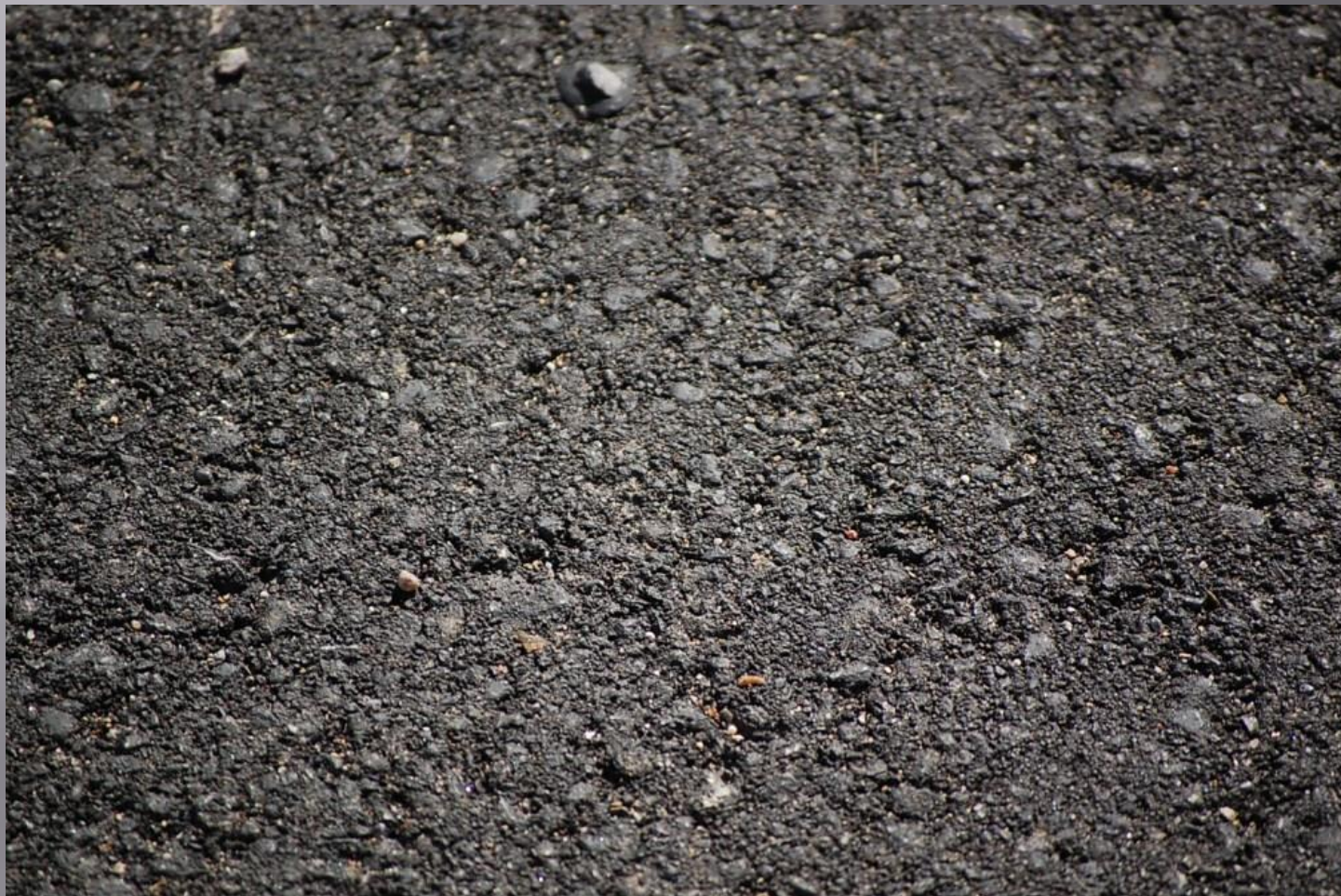
Close-up of rubberized asphalt. Photo by Brian Donnelly TC.
