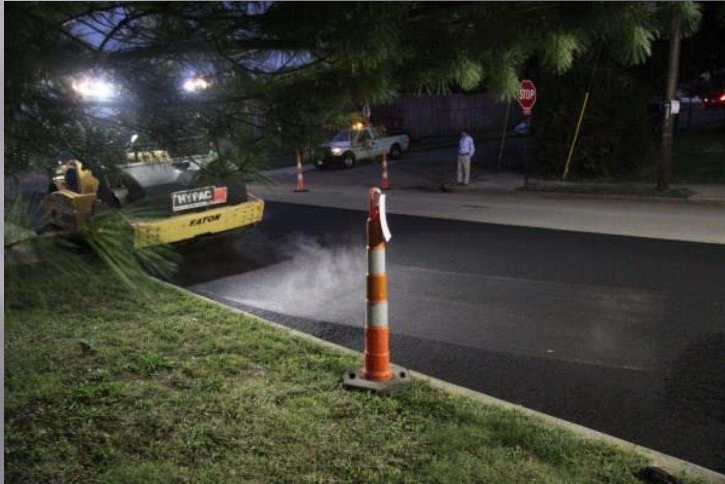
Vibratory roller with view to southeast. Photo by Mark Belshe RPA
