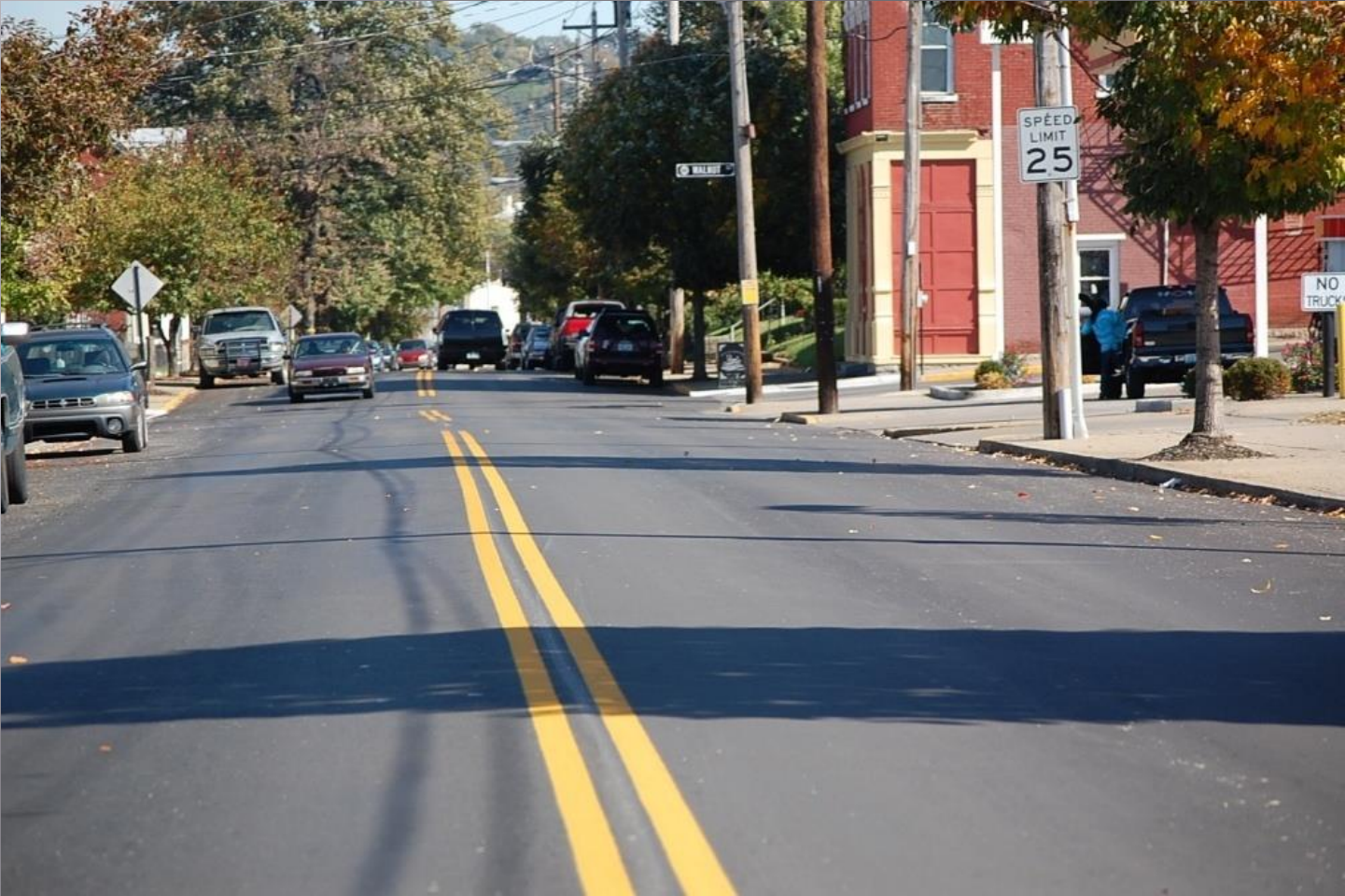
Downtown Dayton KY rubberized and polymer asphalt. Photo by Brian Donnelly TC
