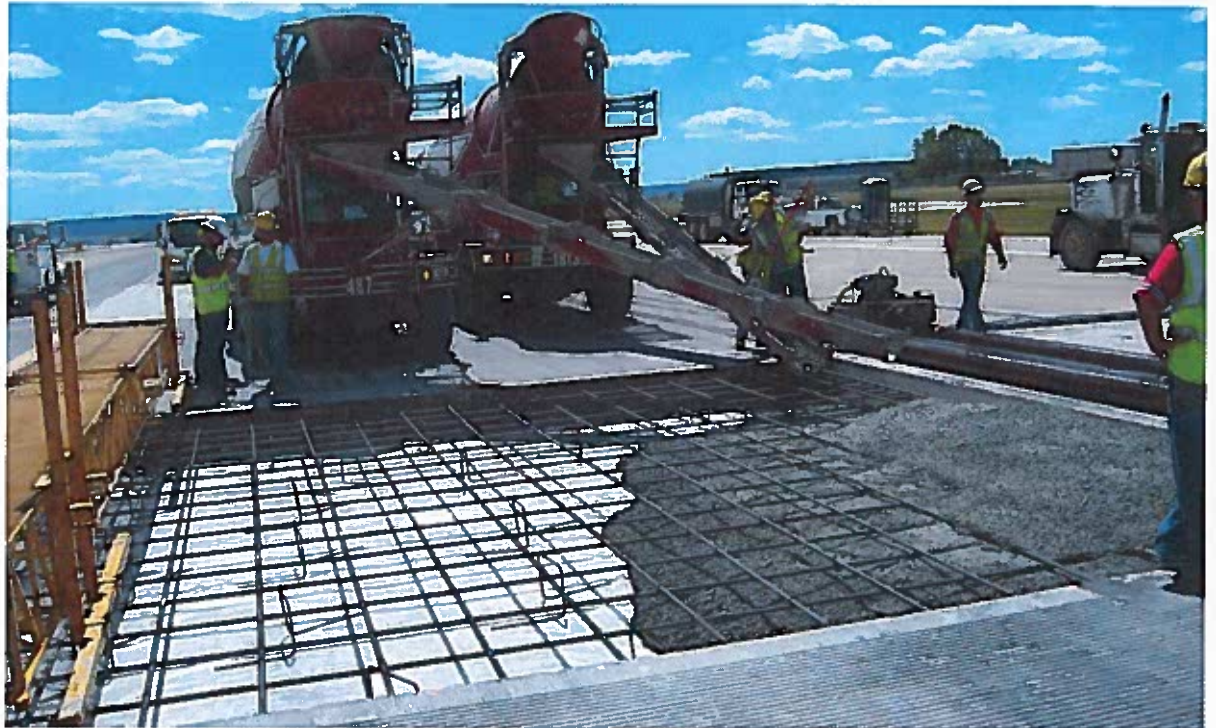
Figure 2. Replacing a concrete panel in Runway 17R-35L at SDF.
