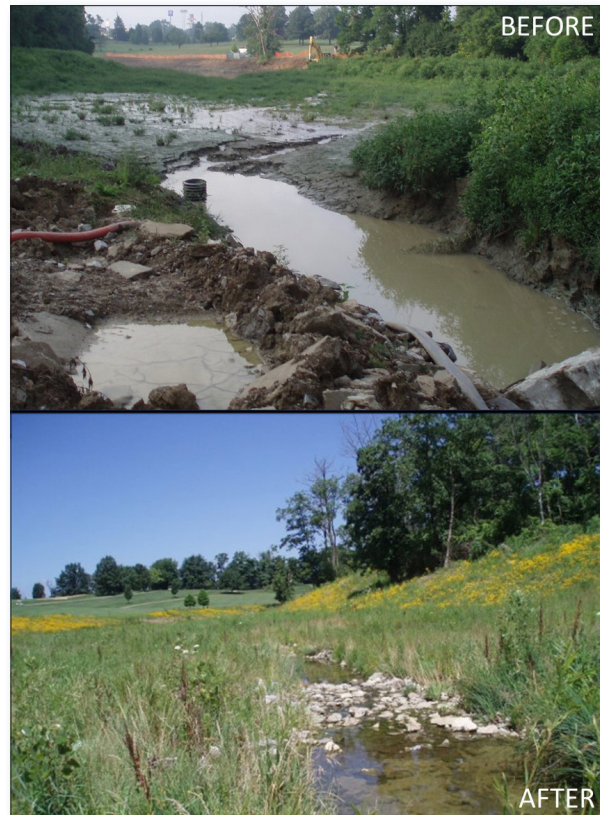
Figure 2. Stream restoration project in Gunpowder Creek watershed.
