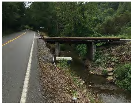
(Left) Metal posts have been inserted to address roadway washout associated with erosion on Sandlick Creek near Dan's Crossing Road. (Right) Roadway washout along Dry Fork near Heartbreak Ridge due to erosion.
