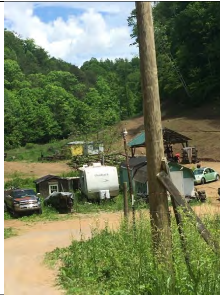
DF#3 focus area of severe erosion
