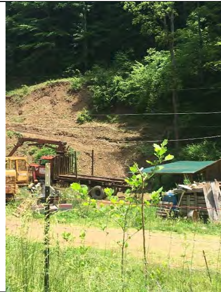
DF#3- focus area of severe erosion
