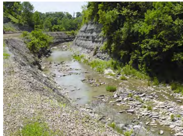
Banklick Creek re-channelized for railroad.
