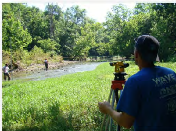
Figure 6-3: Hydromodification surveys measure stream stability and will help to track the impact of stormwater controls on mitigating excess levels of stream erosion
