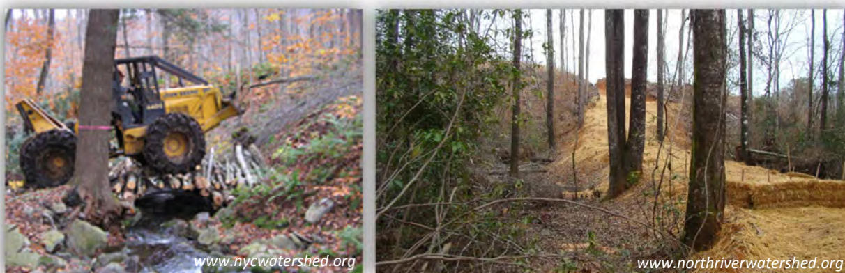
Figure 5-4: Forestry BMPs: Use of a culvert for stream crossing (left) and erosion protection using straw and bales (right)
