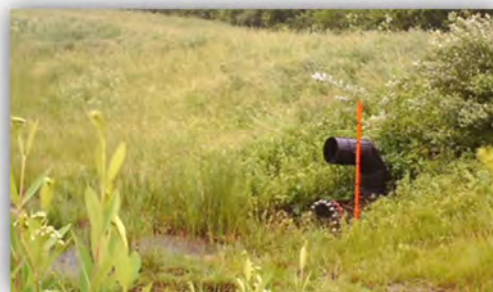
Figure 5-10: Detention basin retrofit technology cost-effectively optimizes excess capacity for downstream channel stability
