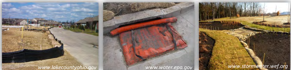
Figure 5-3: Construction BMPs: silt fence (left), inlet protection (middle), and straw wattles (right)
