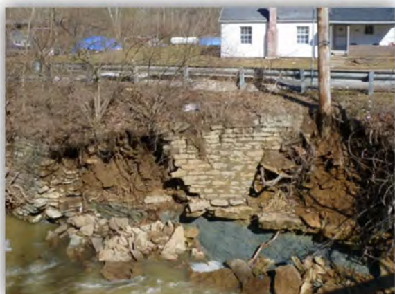
Figure 2-18: Stream disturbances - Collapsing wall on Allen Fork near the confluence with the main branch of Woolper Creek
