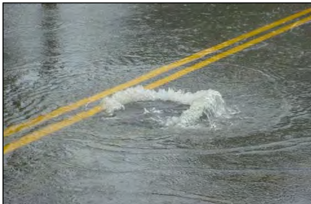
Sanitary Sewer Overflow
