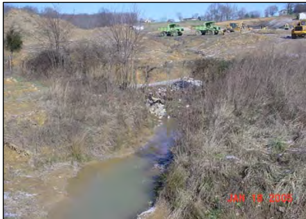
Construction Near Site 23A
