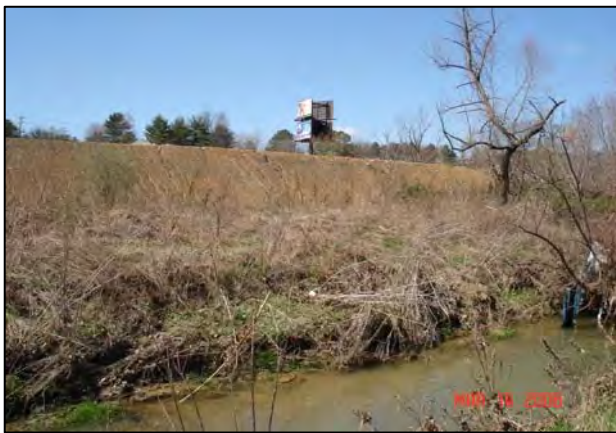
Erosion from Construction Site Adjacent to WWTP Outfall
