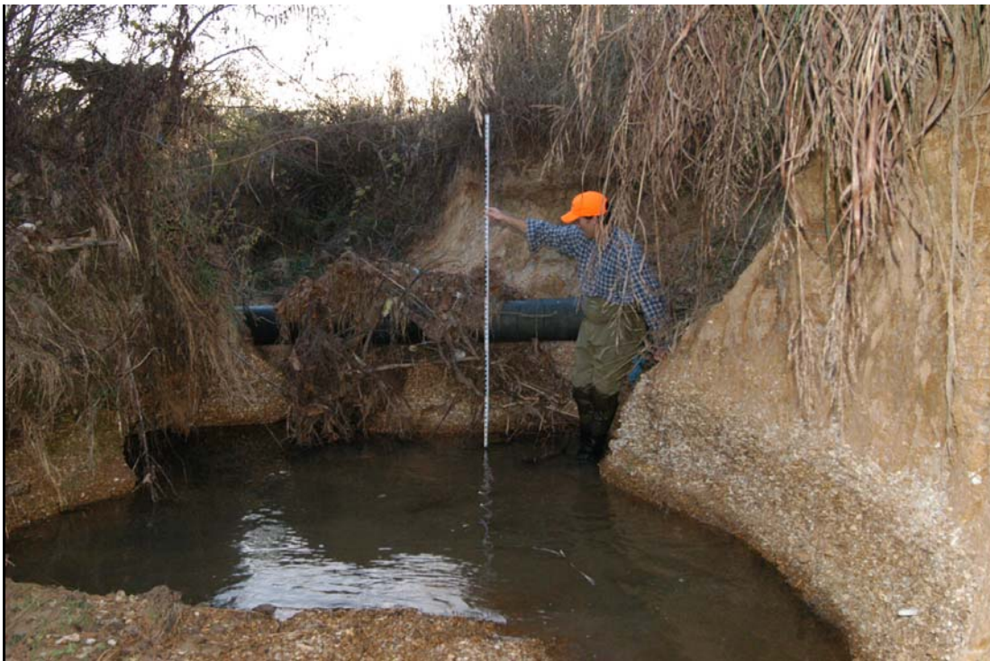
Figure 2.14 Small unnamed headwater tributary of the west fork of Mayfield Creek near the intersection of Kentucky Routes 80 and 384 in Graves County (a) upstream of pipeline and culvert and (b) downstream of pipeline and culvert. Note undermining of waterline in (b).
