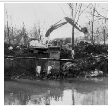
Figure 1.10 Force Main Crossing Beargrass Creek (Louisville MSD, 2007)
