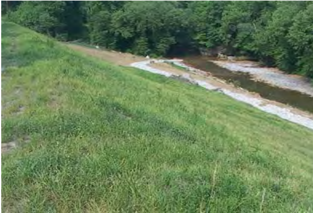
Figure 5. Water Tank Hollow Refuse Area After Reclamation (Phase II) (from Carew et. al., 2003)
