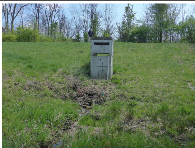
Detention Basin Outlet Control Structure
