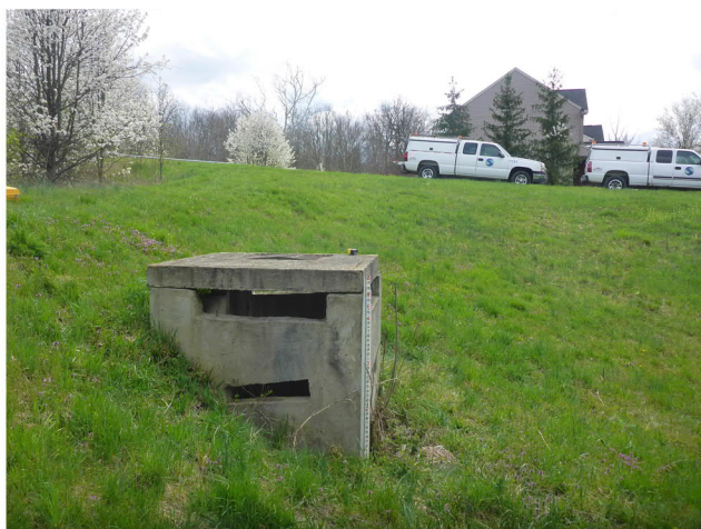
Detention Basin Outlet Control Structure
