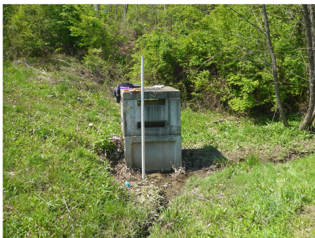
Detention Basin Outlet Control Structure
