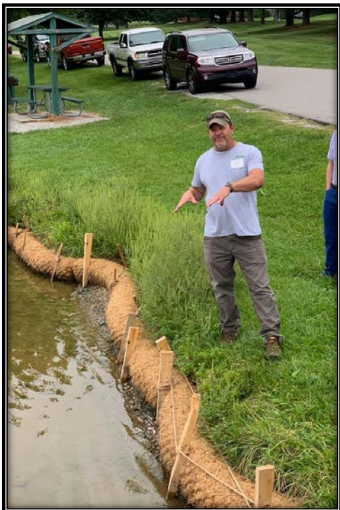
Figure 2.7.3 Shore Stabilization at Camp Ernst Lake
