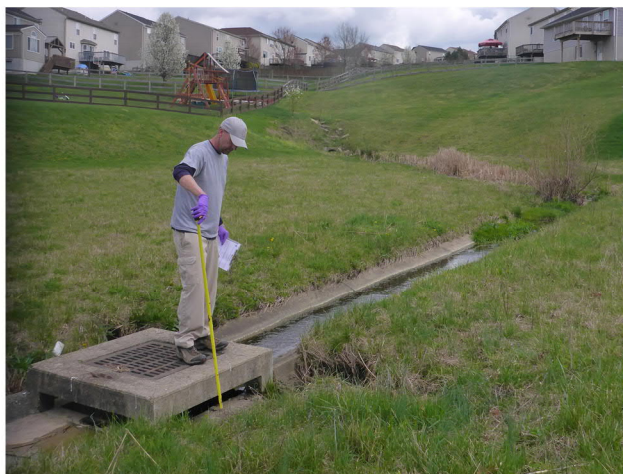
Outlet Control Structure at Bottom of Basin
