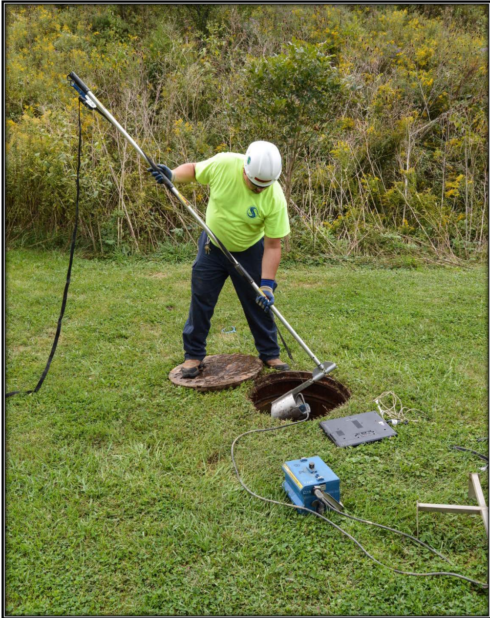
Figure 2.4.2: SD1 performing a sanitary structure inspection
