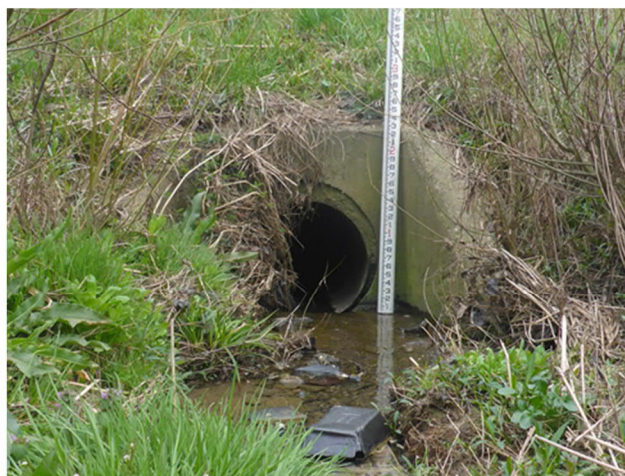
“Low-Flow” Pipe at Basin Bottom
