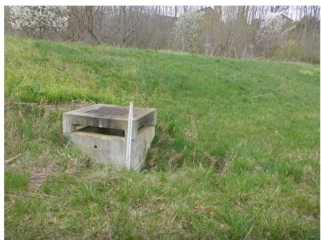
Outlet Control Structure on Side Slope of Basin
