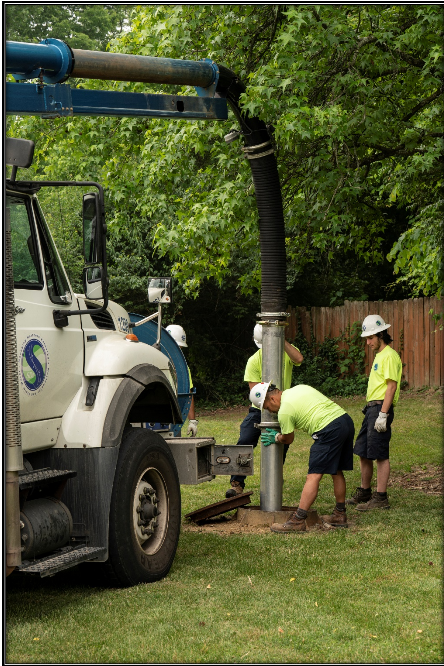
Figure 2.5.2: SD1 performing sewer maintenance
