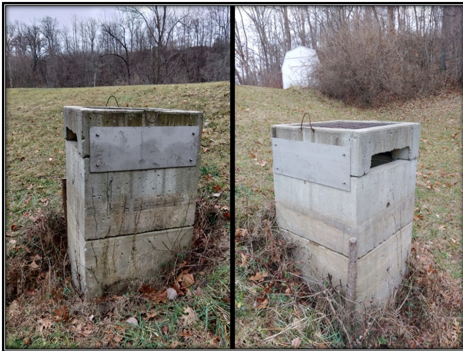
Figure 2.6.3 Detention basin retrofit with plates on outlet control structure
