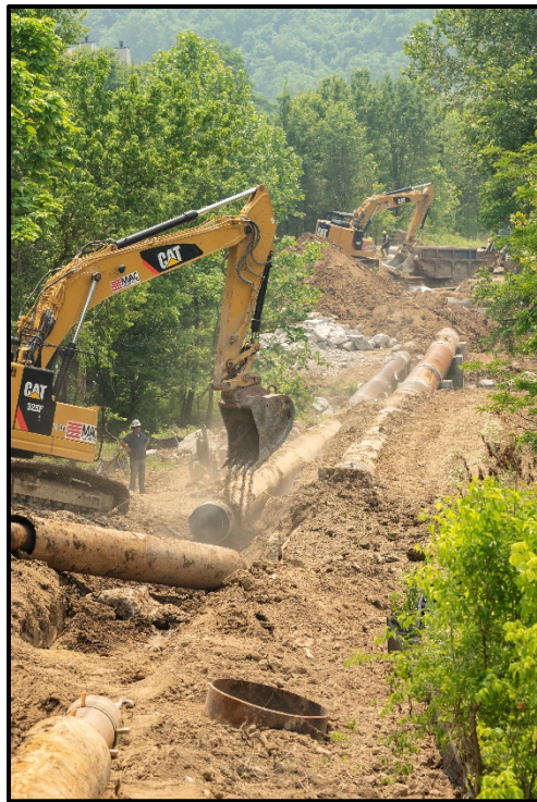
Figure 2.4.2 and 2.1.3: Installation of the LRS conveyance piping
