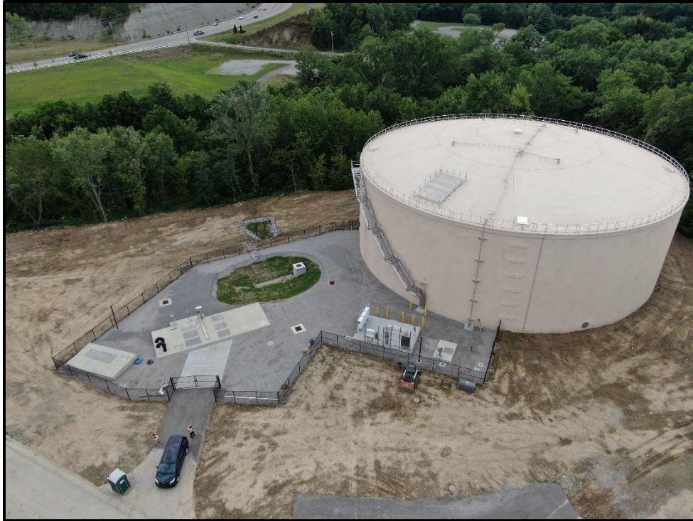
Figure 2.3.2: The completed LRS EQ Tank
