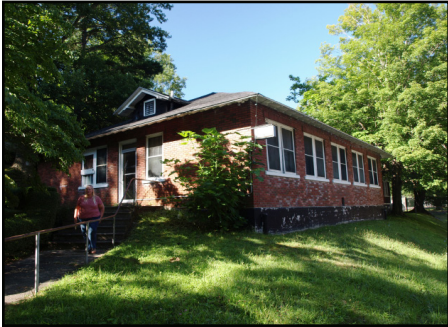
Former clinic in Benham
