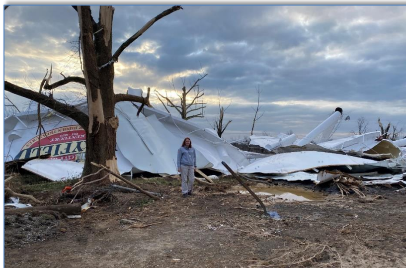
Shannon McLeary, DOW/ERT Incident Commander, standing in front of destroyed Mayfield 500,000 gallon water tank
