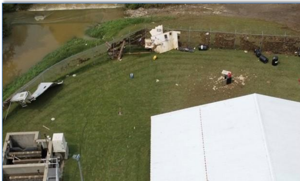
Remains of chemical storage building in fence debris.
