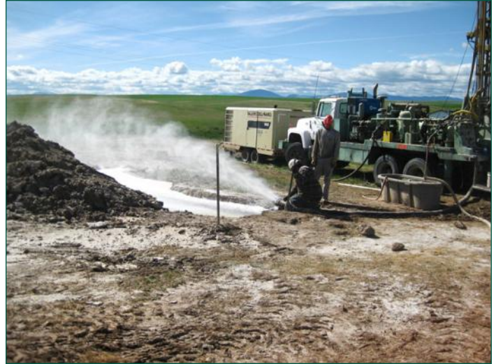
New well drilled for Sand Coulee.
