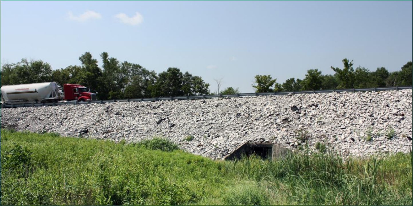
Completed road stabilization project.
