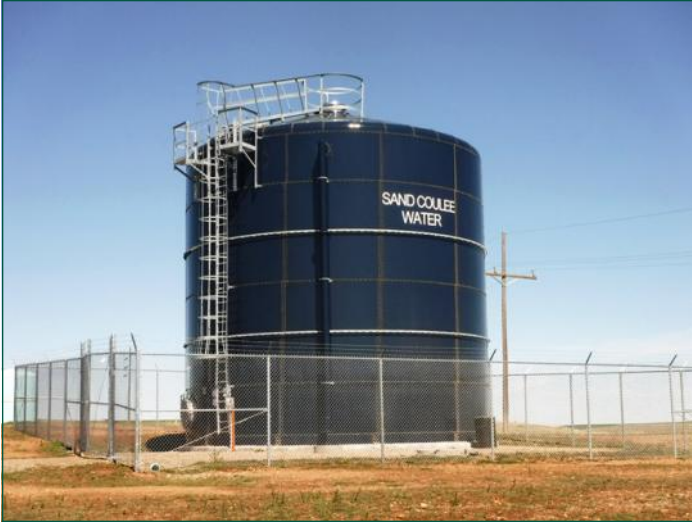
New water storage tank for the town of Sand Coulee.
