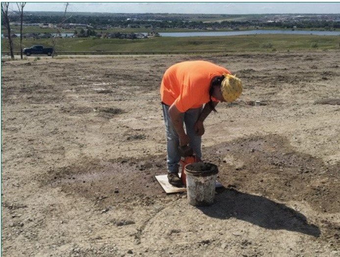
A material tester conducting a slump test in Williston 2019.
