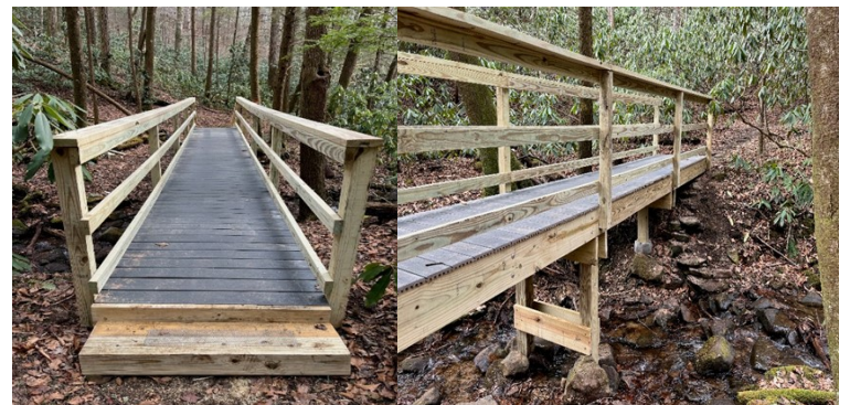
New footbridge installed at Blanton SNP
